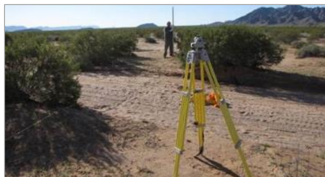
Figure 3.2: Road elevation measurements being taken using California rod and auto-level.
