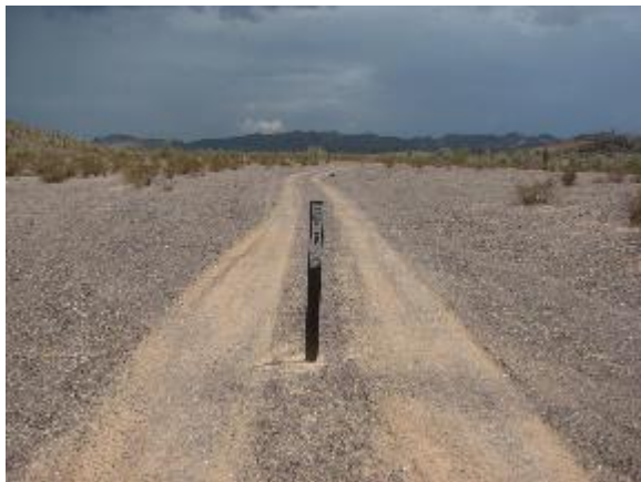
Figure 6.1: Example of a road closure sign.
