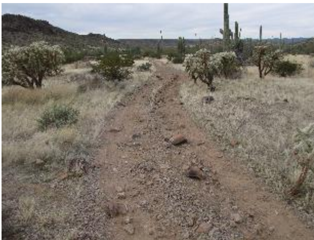
Figure 5.1: Unimproved public access road.
