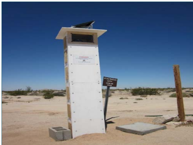
Figure 3.3: Observation tower house cameras that monitor human activity and erosion.
